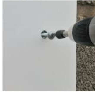
C. Position fixture, tighten bolt into shield
