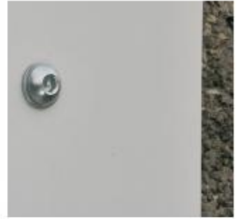
D. Secure removable fixing
