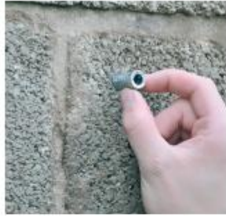
B. Insert Anchor shield
